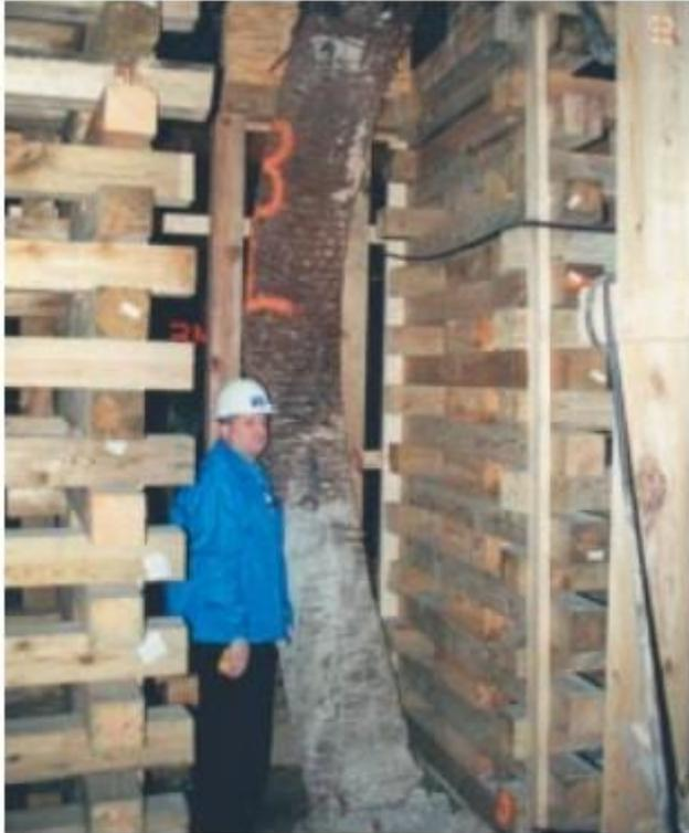
Figure 5.20 Column 3L with large deformation and discrete hinges
